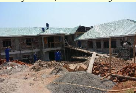
The multi-million building at Kibiito, Kabarole district
