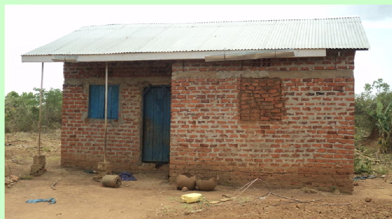
The new family house built with savings from their group
